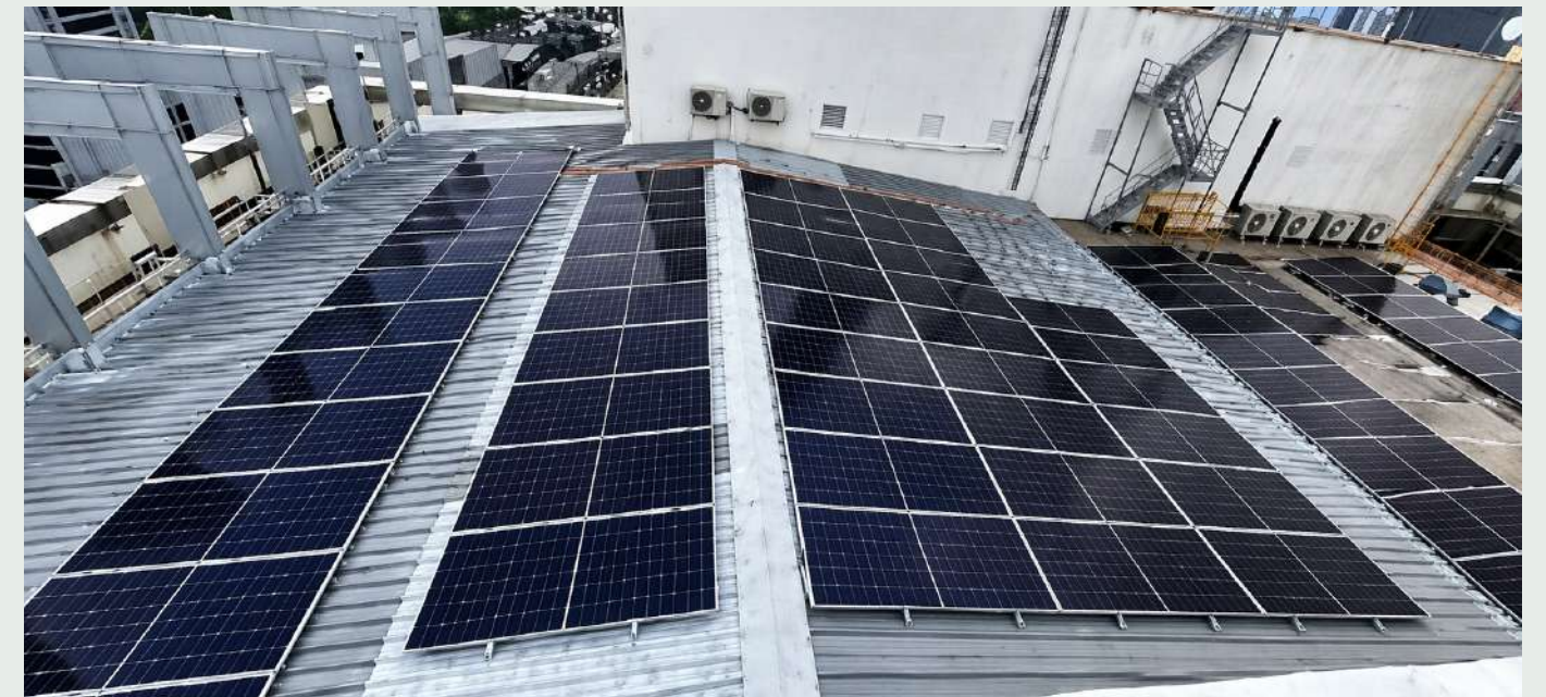
A rooftop solar panel system was installed at Kenanga Tower to increase the share of electricity sourced from renewable energy, supporting our efforts to decarbonise Scope 2 emissions under the Decarbonisation Roadmap.
