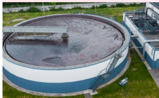
Water treatment plant in Linshu
