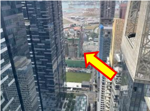
Construction Progress of W Residence
